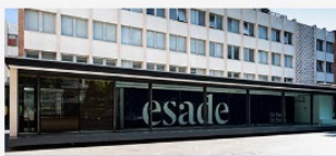
Building 1 - Av. Pedralbes
